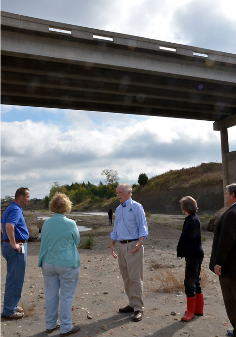
Tom Taylor, Executive Director of Upper Trinity Regional Water District (center) and Ladonia Mayor Jan Cooper (second from right), answer questions from reporters as the groups stands in the river channel 60 feet below the Hwy. 34 bridge. While this existing bridge would be 50-feet underwater when Lake Ralph Hall is full, an elevated bridge will cross the lake at this same location.
